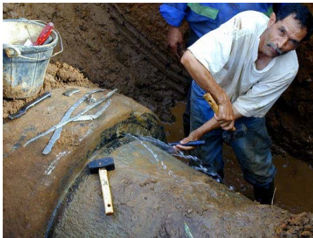
Repairing a leak found using Sahara
